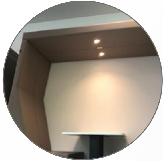
Lights with PIR sensor
